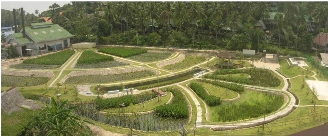
Fig. 3. The 'butterfly' wastewater treatment system at Koh Phi Phi Don is planted with beautiful flowers, such as Cannae and Heliconia to make it aesthetically pleasing.
